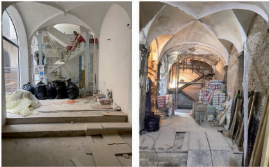
ENTRANCE HALL BEFORE DURING THE RESTORATION WORKS
